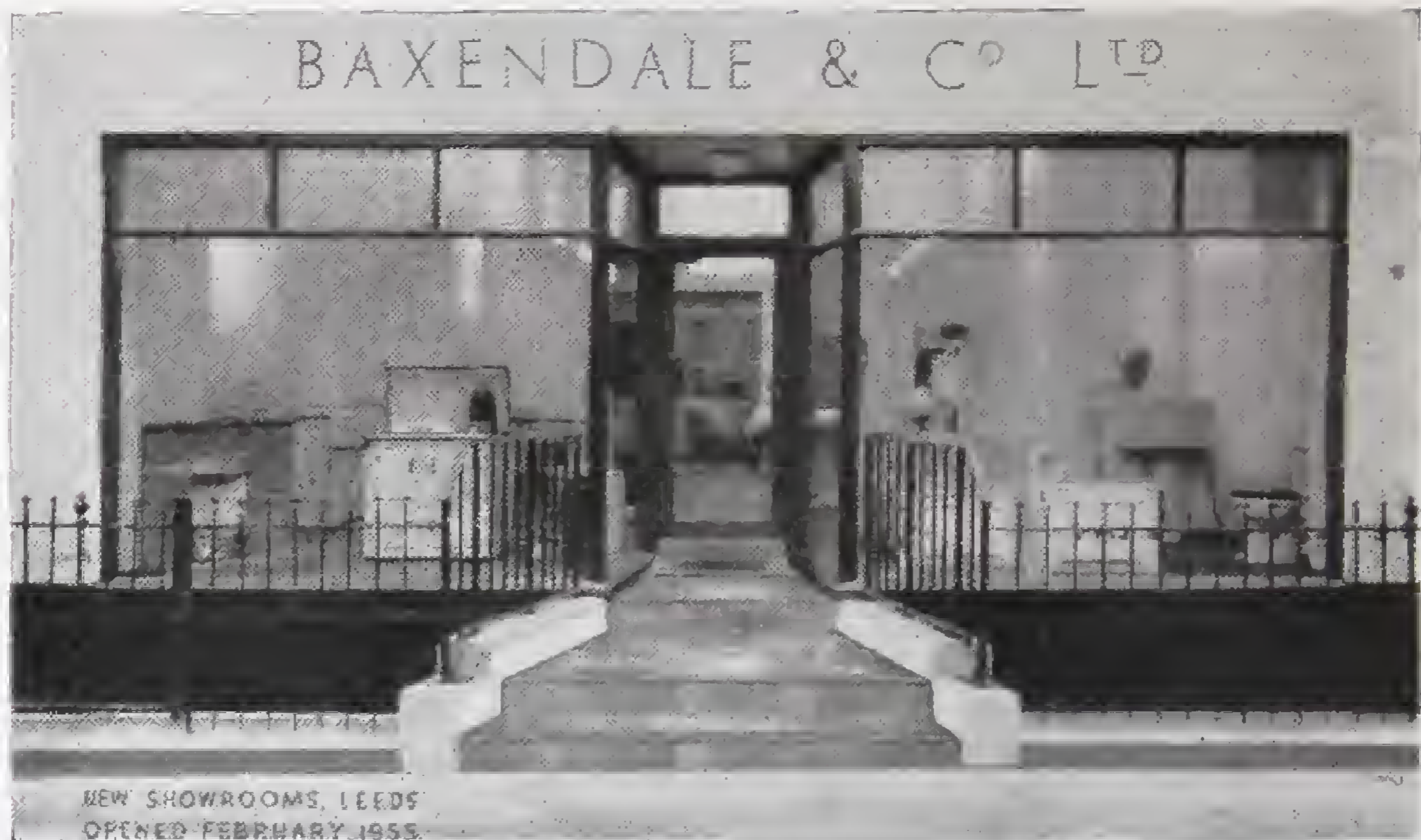
Shop Fronts with raised or incised lettering on facias—including Glass or Vitrolite for Fascias, Transoms, Stall Risers, and Pilasters.
